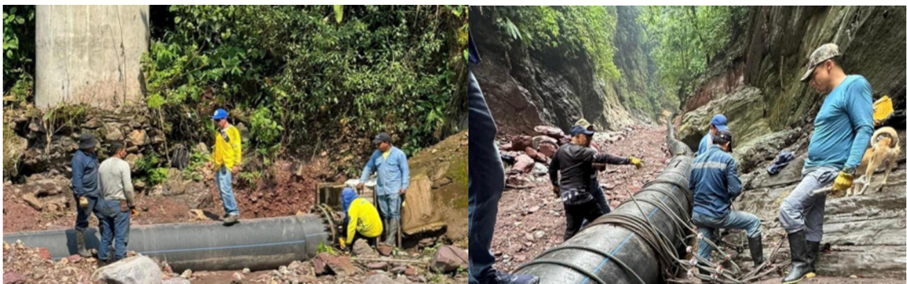
Figure 4. Repairs to the adduction system in Quebrada la Honda
